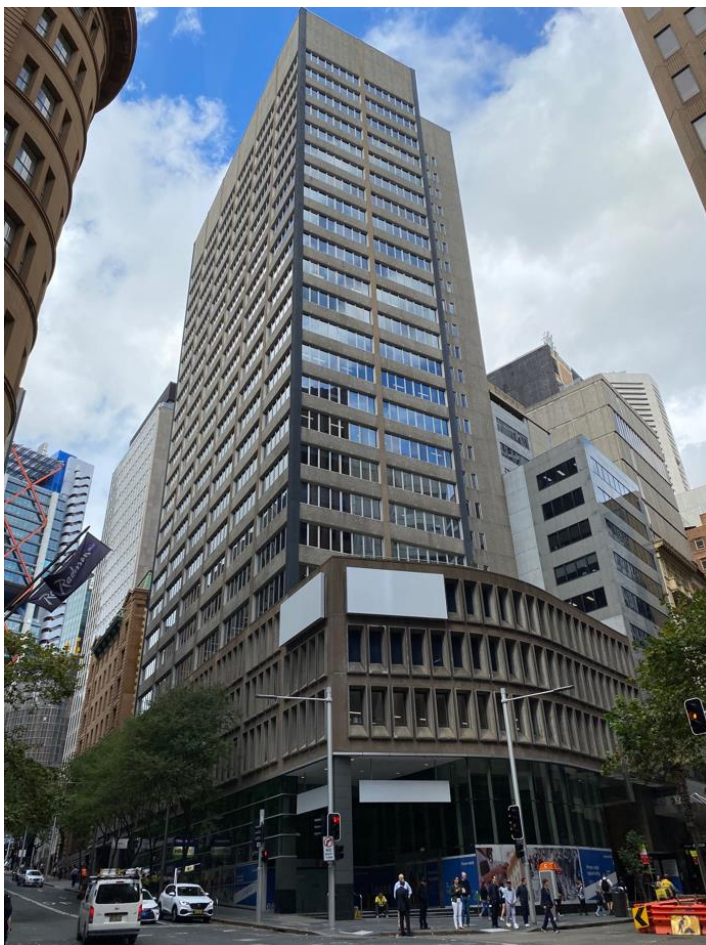
Figure 6: East of the site, looking the south-east corner of Hunter and Pitt Streets
